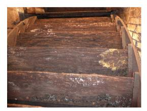
There are 36 'buckets', each formed by three timbers - the sole board, the riser, and the ladle board. To keep the mill running, we have taken on the huge task of replacing all 108 boards before we open again to the public on 26th March.
